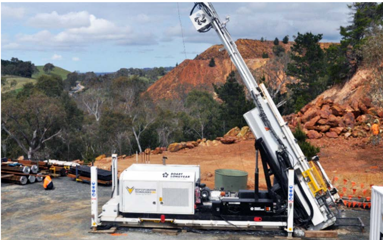
Figure 2 Boart Longyear 4200 drilling rig on site at the Brukunga Mine. (Photo 409690)
