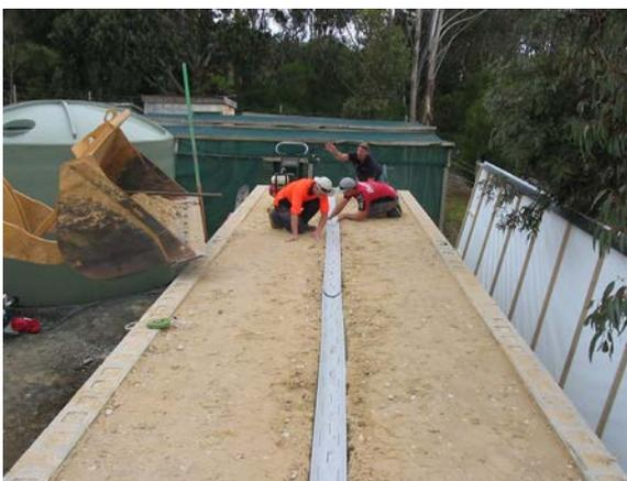
*Construction of the 100 tonne trial for the proposed Brukunga saturated co-disposed mine waste model. (Photo 413489)*
