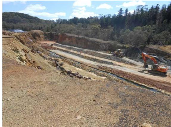
*Construction of the geotechnical remediation trial for the proposed Brukunga saturated co-disposed mine waste model. (Photo 413490)*
