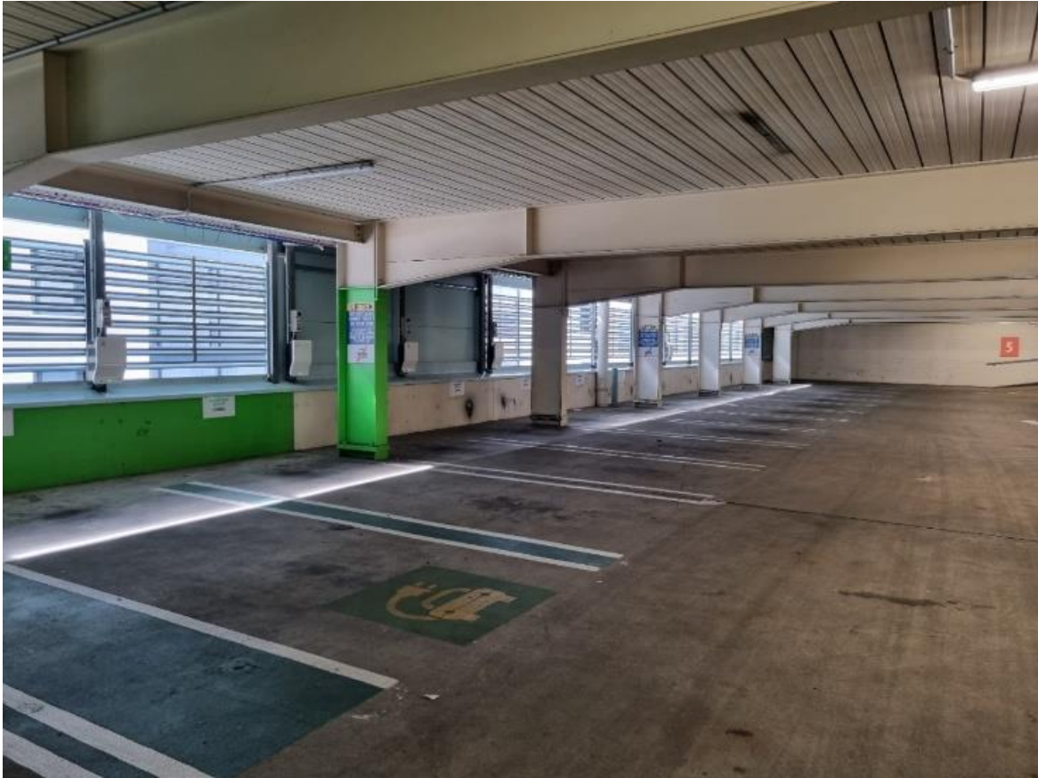
Figure 2: EVlink Smart Wallbox Chargers (7.4kW – T2 – RFID) at Wyatt UPark
