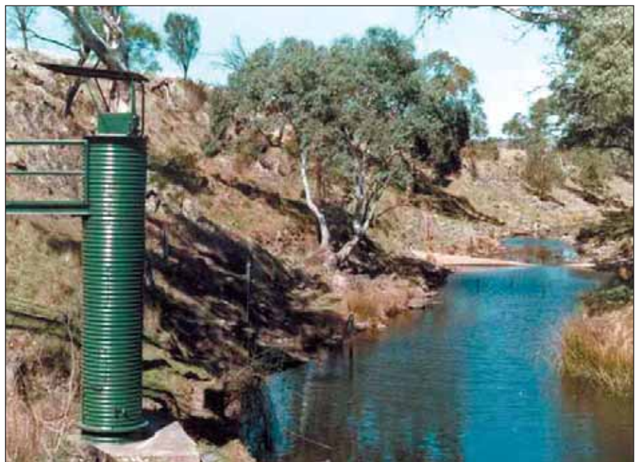
Plate 5.10 Bremer River stream gauging station site
