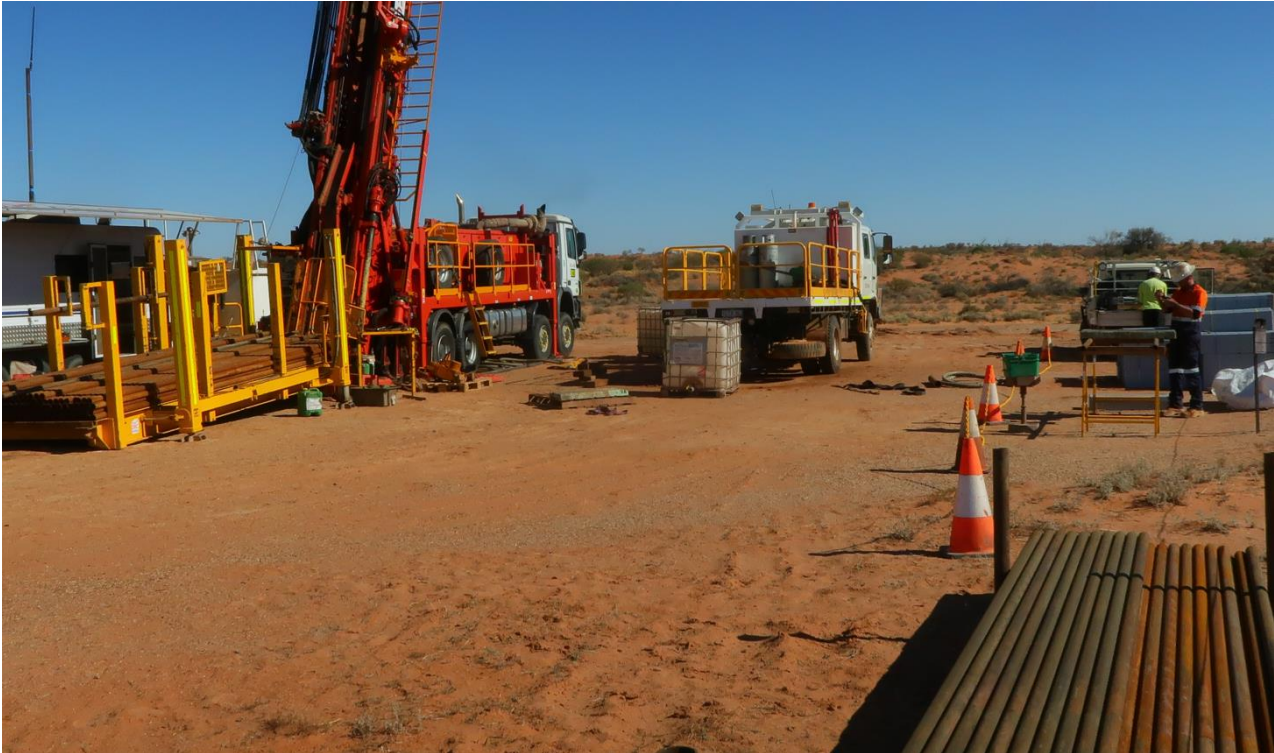
Photo 4. Example of drill site set up and equipment. The photograph of typical drill site showing (L to R) rod rack/sloop (on a hydraulic powered flatbed truck platform), driller office caravan drill rig, support truck, core presentation and processing area.
