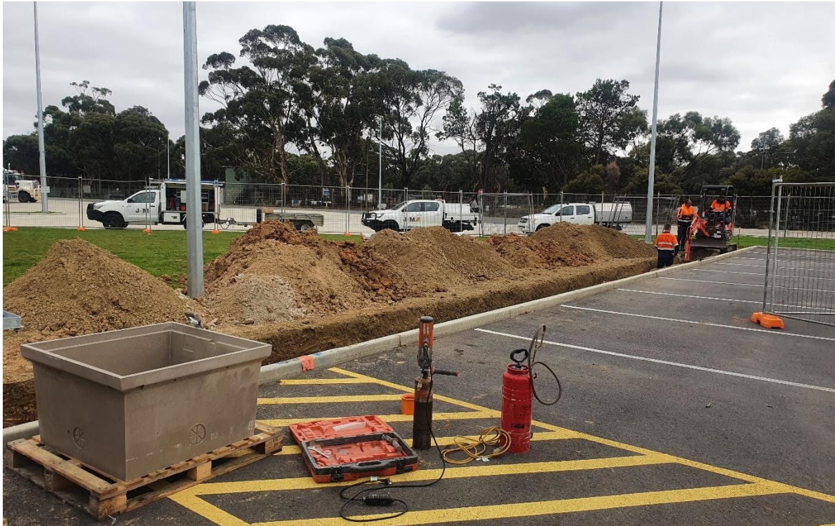
Figure 4. Civil Works Construction
