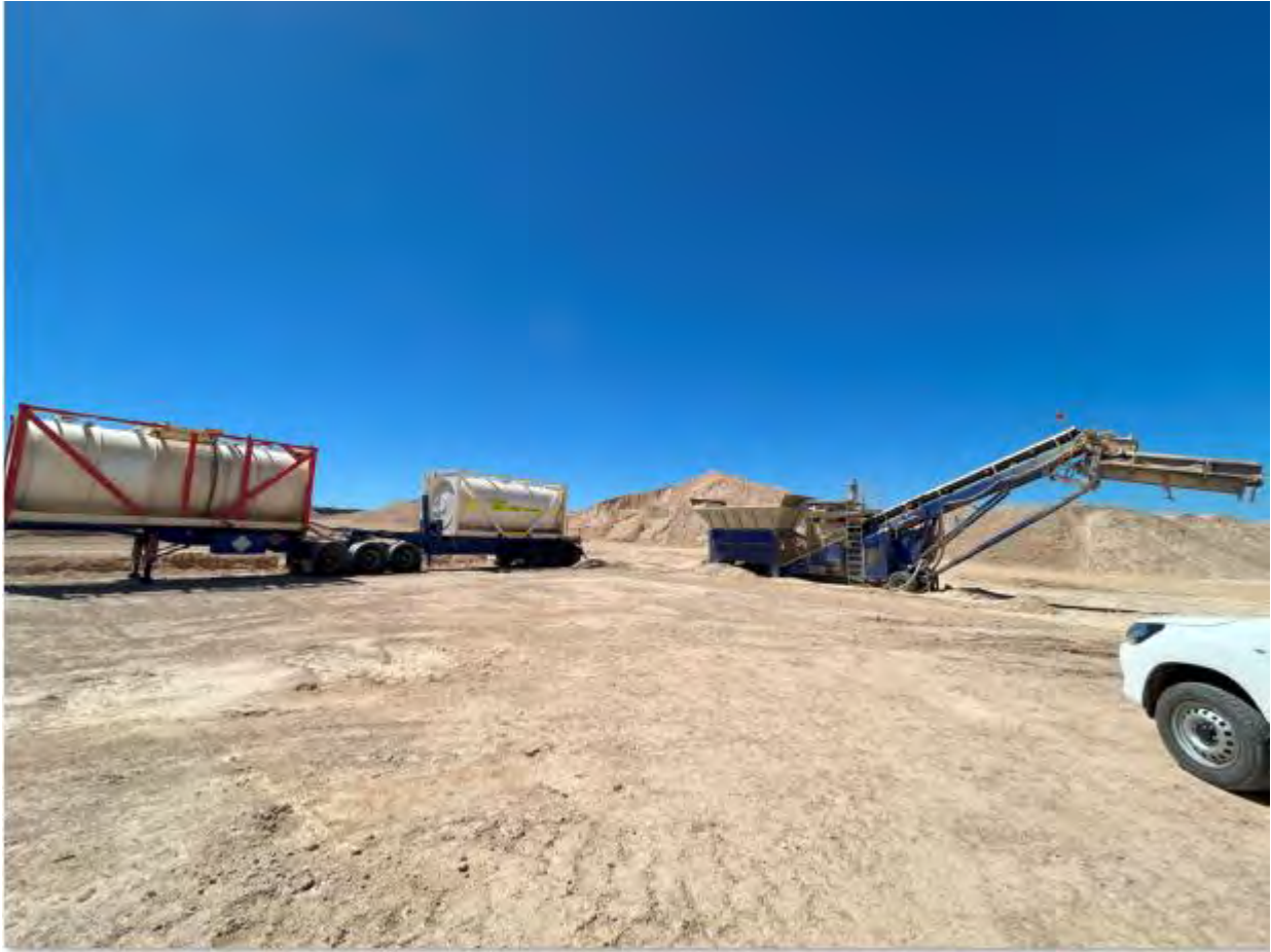
Photo 1 - Crushing and Screening Operations February 2024
