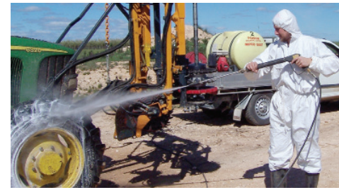
Decontaminate wheels and steering
