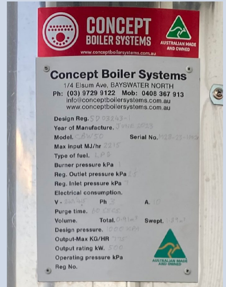
Figure 2 – Example of Type B appliance Markings
