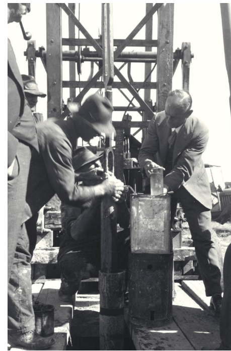
Testing gas in Ramsay Oil Bore, 1931
