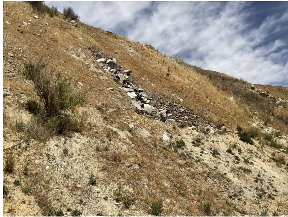
Surface Water: Rock catchment drainage on quarry walls to prevent erosion.
