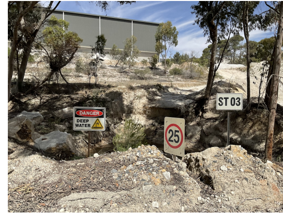
Surface Water: Sediment trap with public safety signage.
