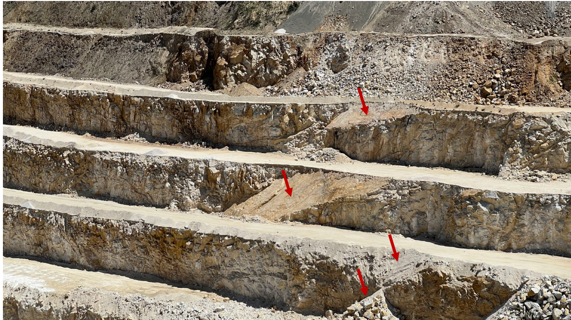
Figure 12: Central west wall slipperybacks, planar and wedge formation.
