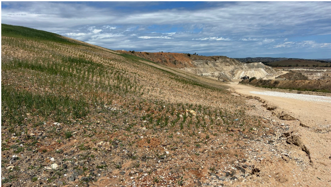
Figure 16: Eastern rehabilitation mound structure toe.
