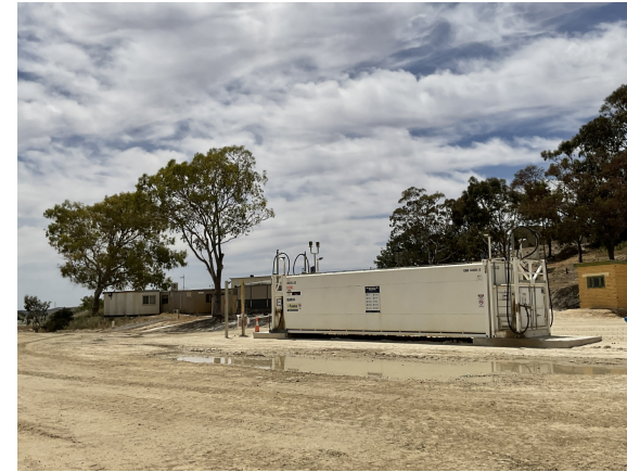
Hydrocarbons: Self bunded diesel tank.
