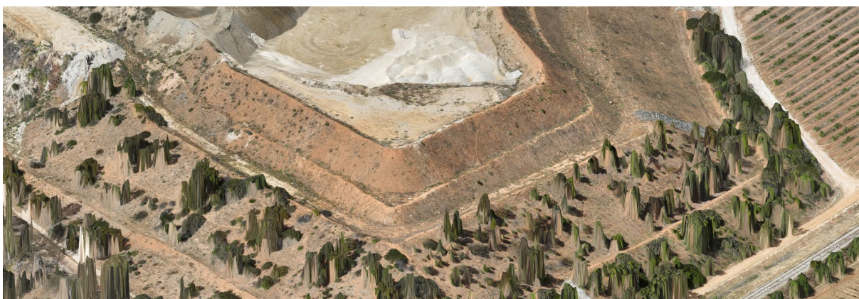
Figure 19: West overburden dump.
