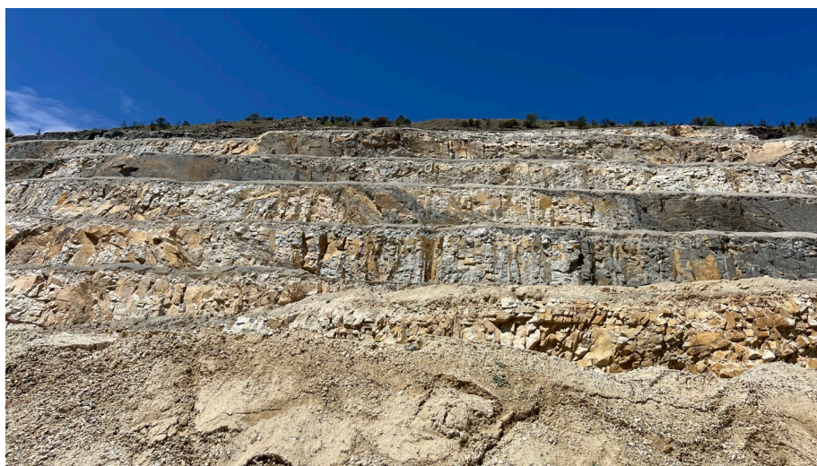
Figure 15: Central east wall highly jointed and fractured rock mass.
