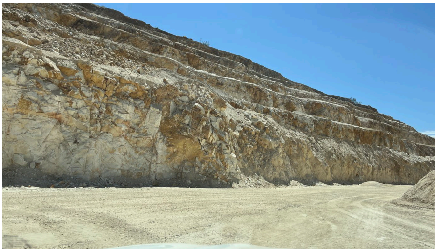
Figure 14: Southwest west wall highly jointed and fractured rock mass.
