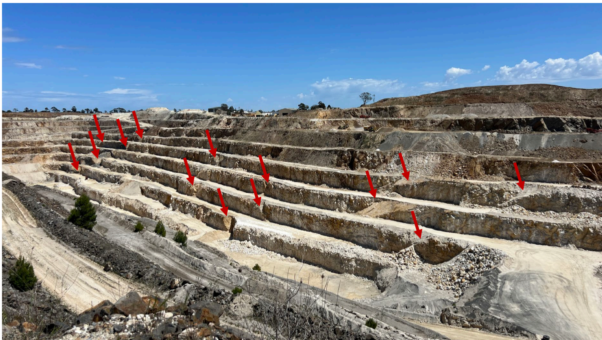
Figure 11: High occurrence of wedge failure in the west wall.
