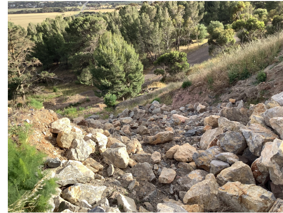
Erosion, Sediment and Stormwater Management: Surface water bund.
