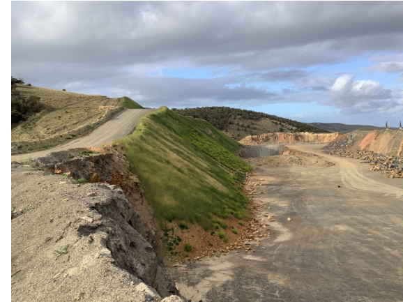
Erosion, Sediment and Stormwater Management: Haul road sloping / bunding well-vegetated to prevent erosion.
