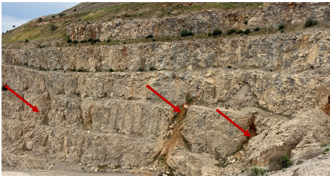
Figure 14: Highwall adjacent to the main haul ramp to the upper level and immediately behind the plant.
