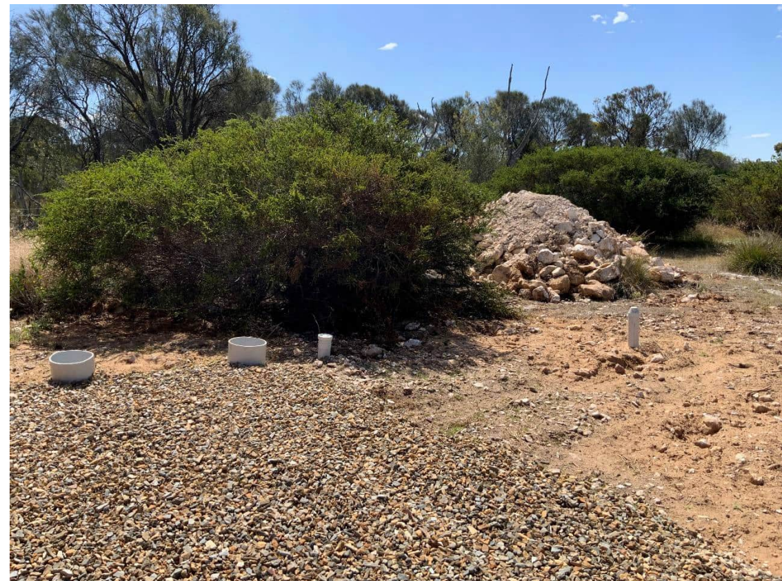
Photo 15: Photo – Septic tank installed
