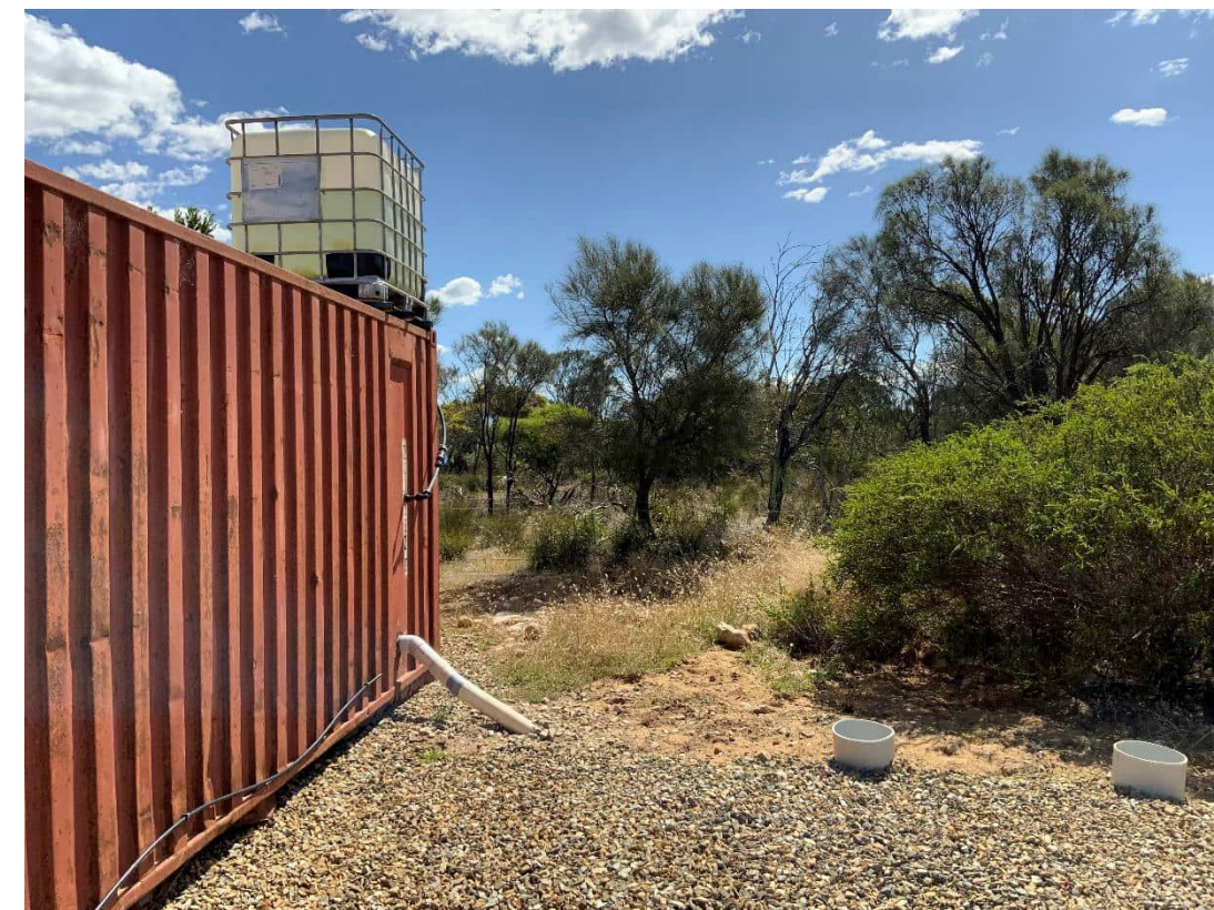
Photo 17: Photo - Septic tank installed
