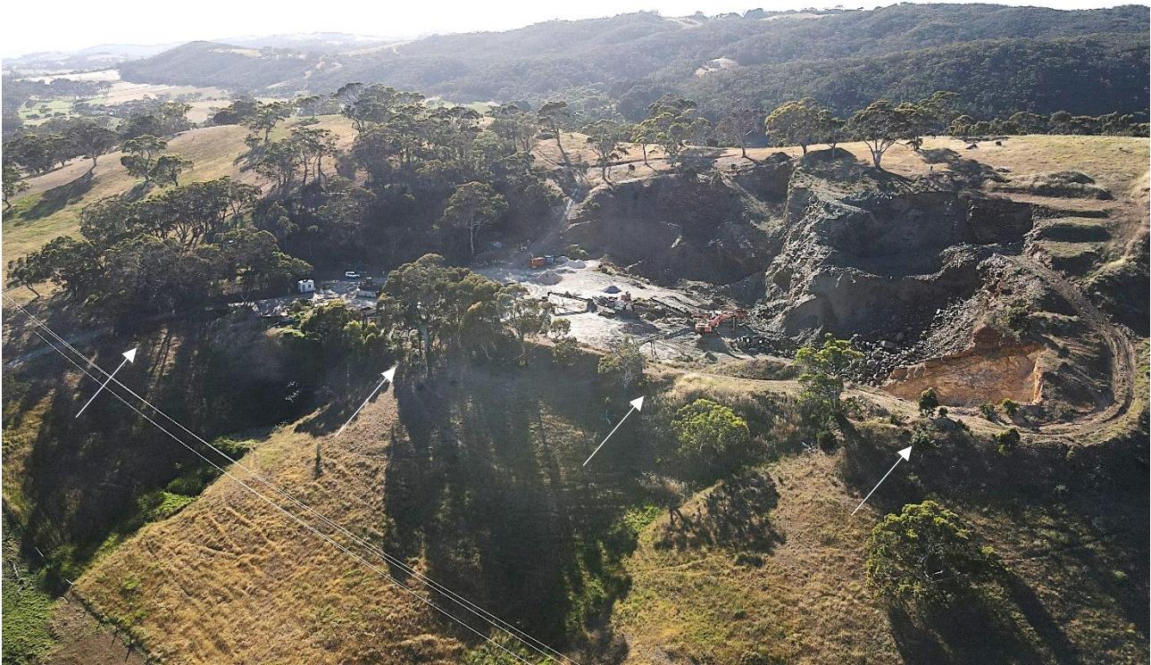
Plate 5 – The partial tree screen along the northern side of quarry
