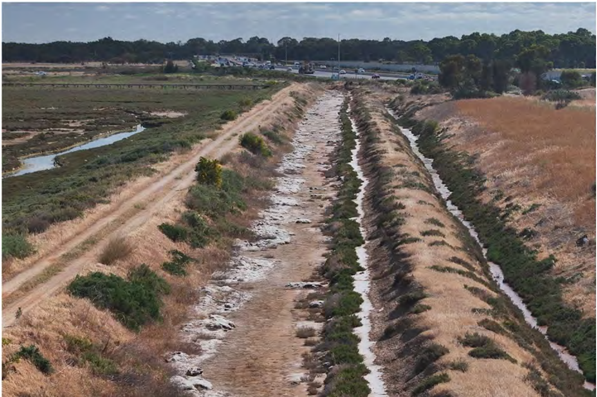
Photo 12: View north at existing open channel near PA12, Council drain to right
