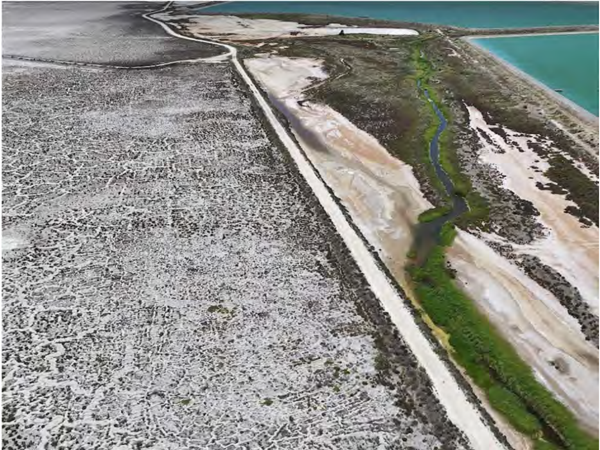
Photo 5: View north at PA9 and PA8
