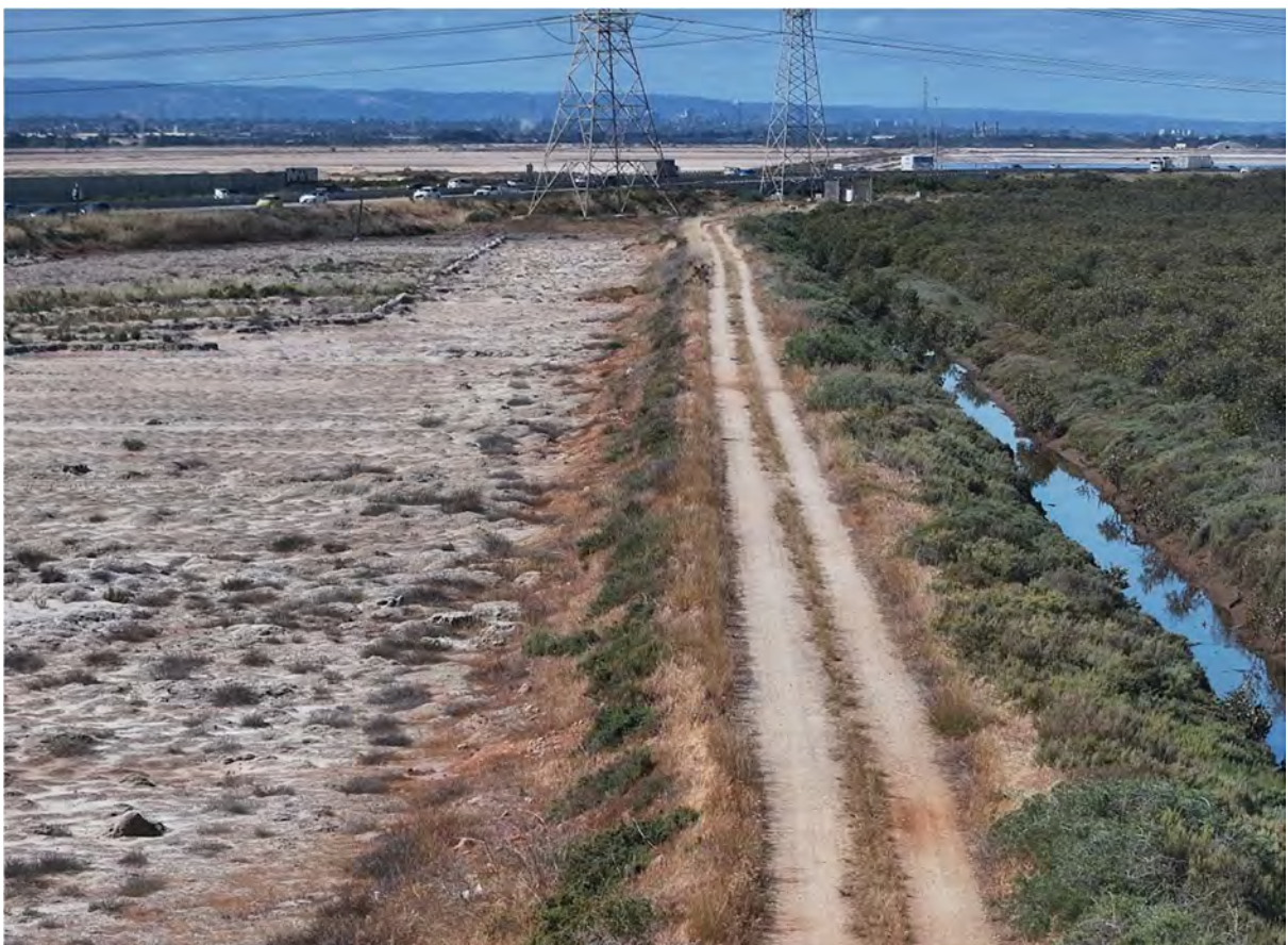
Photo 14: View south at PA12 and Peter's Peak pumpstation
