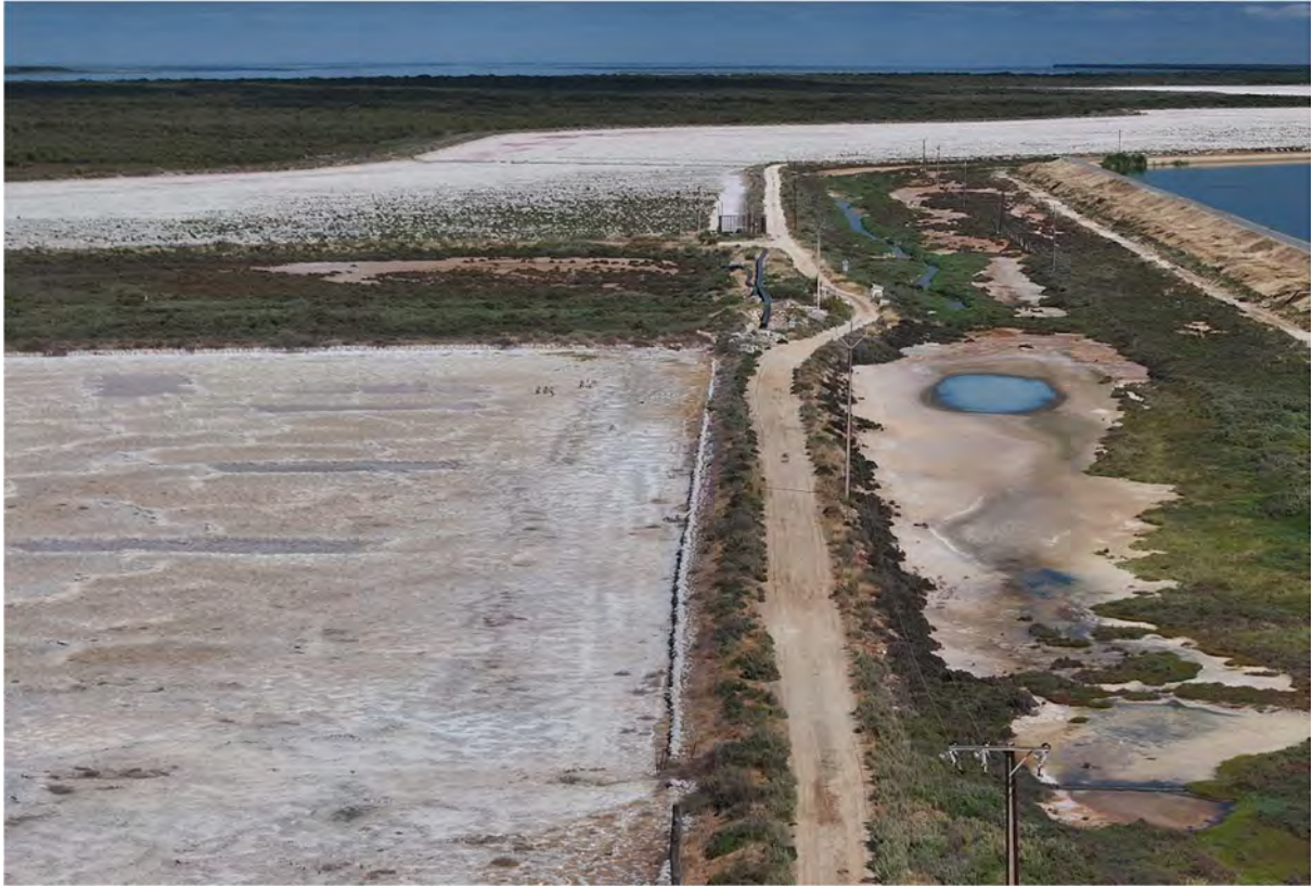
Photo 7: View north at PA10 and PA9 with 1 st Council drain crossover
