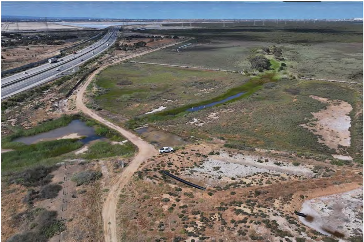
Photo 10: View south at Little Para River crossing and channel to PA12
