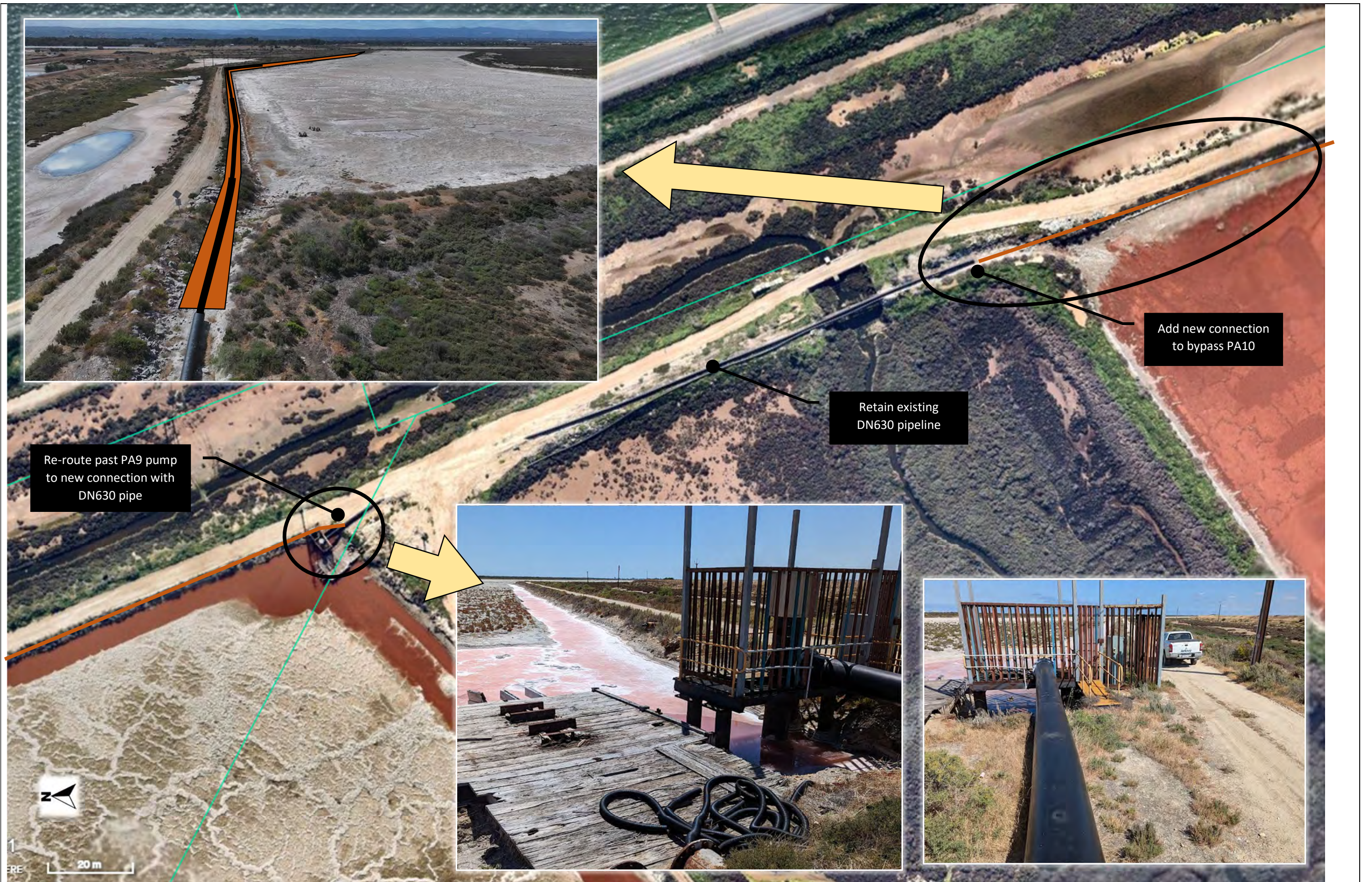
Figure 3: PA9 pump and Helps Road Drain crossing
