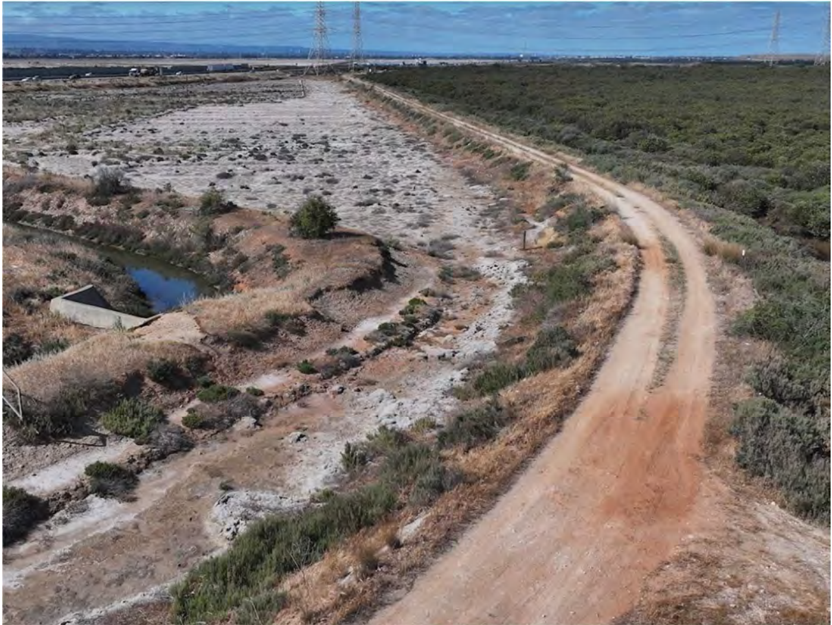
Photo 13: View south at channel outfall to PA12
