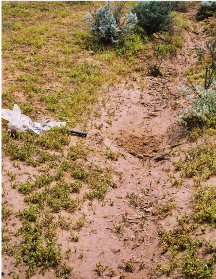
Plate 3.2 Fine-Grained Material Washed From Stockpile Area
