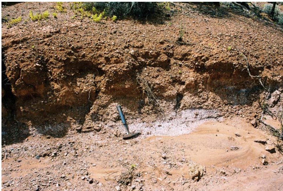
Plate 3.3 White Efflorescence in Drainage Channel South of WRD
