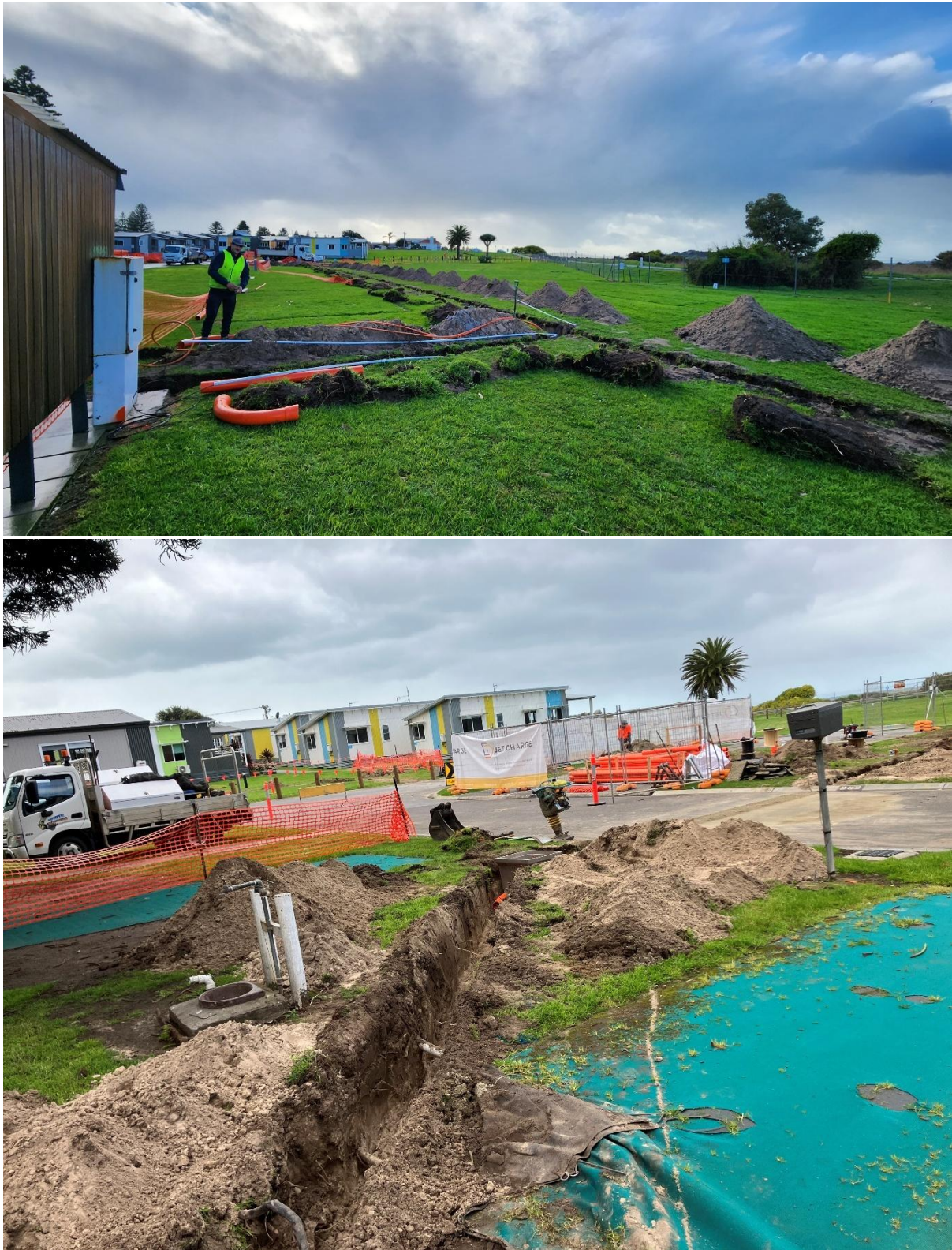
Figure 6. Civil Works & Trenching
