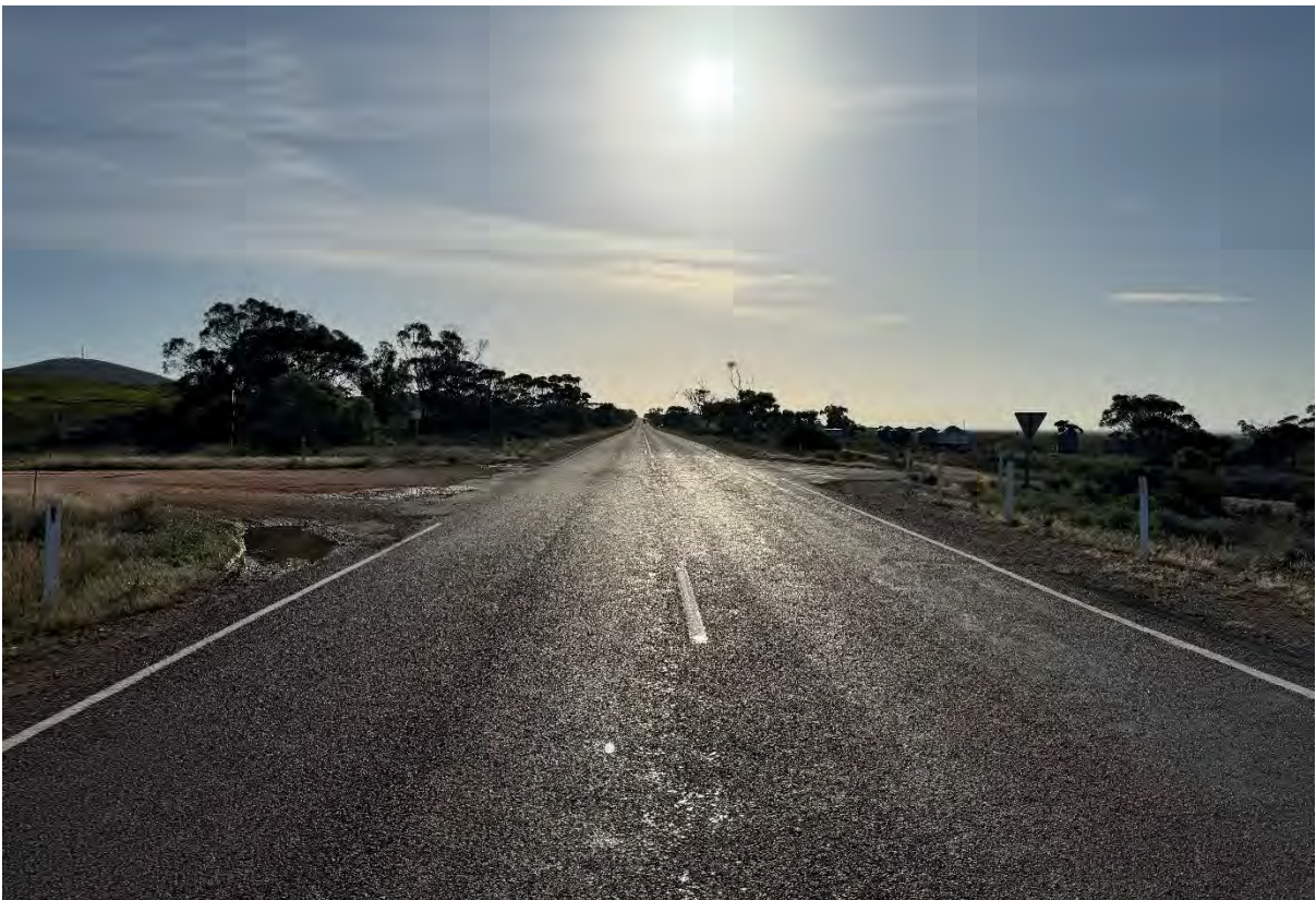
Figure 17: View from Lincoln Highway intersection looking in the direction of Cowell.
