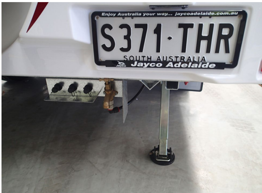
Figure E 5: Non-compliant electrical installation caused an electric shock on this tap
