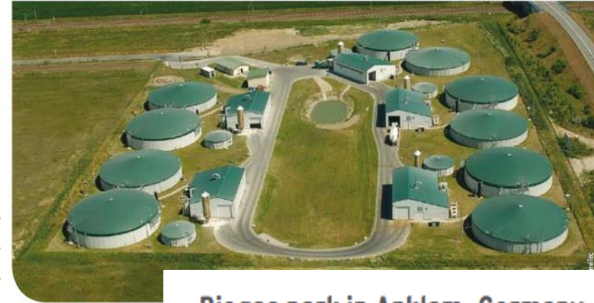
Biogas park in Anklam, Germany
